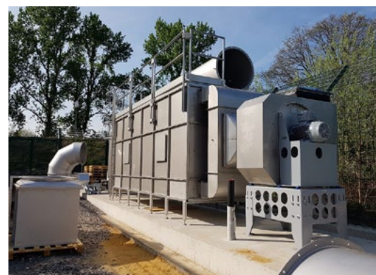
EMSCHER LIPPE Emscher DE Sewage network 50 km 390 000 m 3 /h > 95% odor reduction ColdOx® system x 18
