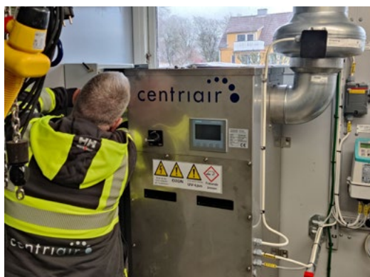
BORÅS Borås SE 20m next to public beach 150 m 3 /h > 95% odor reduction ColdOx® system
