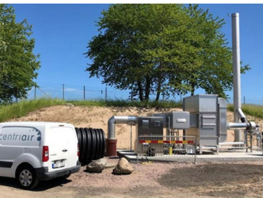
SKÖVDE Skövde SE Septic tank sludge 4200 m 3 /h 21 173 to 30 ou/m 3 > 97,7-99,5 % reduct. ColdOx® System
