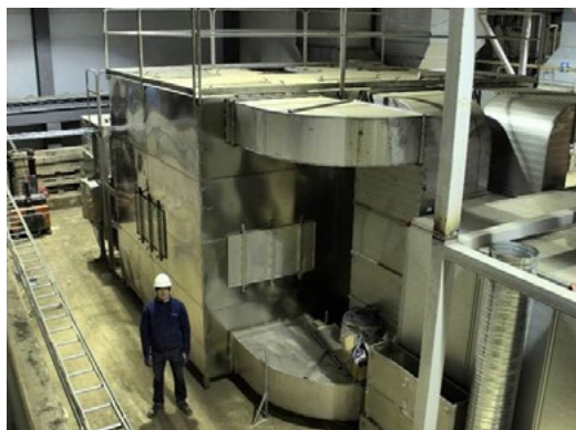
RENOVA Göteborg SE Organic waste 72 000 m 3 /h > 95% odor reduction ColdOx® x 3
