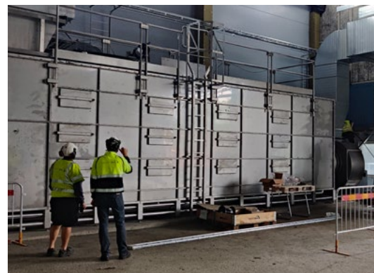
RENOVA Göteborg SE Hazardous waste 67 000 m 3 /h > 95% odor reduction ColdOx® system
