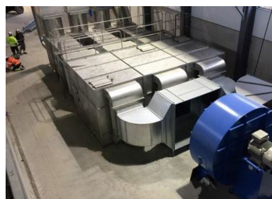
HEM Halmstad SE Solid Waste 90 000 m 3 /h > 95% odor reduction Filtration+ColdOx®
