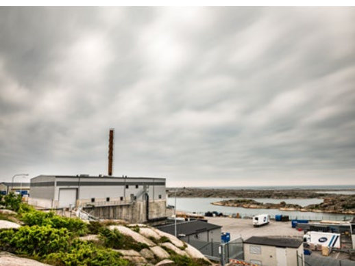
RENA HAV Sotenäs SE Biogas production & treatment plant 30 000 m 3 /h > 95% odor reduction ColdOx® system, SulphaRed bi-flow
