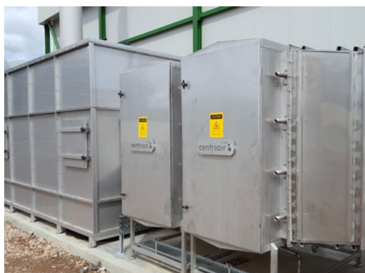
BIOCONSTRUCT Hartpool UK Twin Biogas Plants 20 000 m 3 /h > 97% odor reduction ColdOx® system
